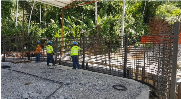
Fixing steel reinforcement cages for invert
