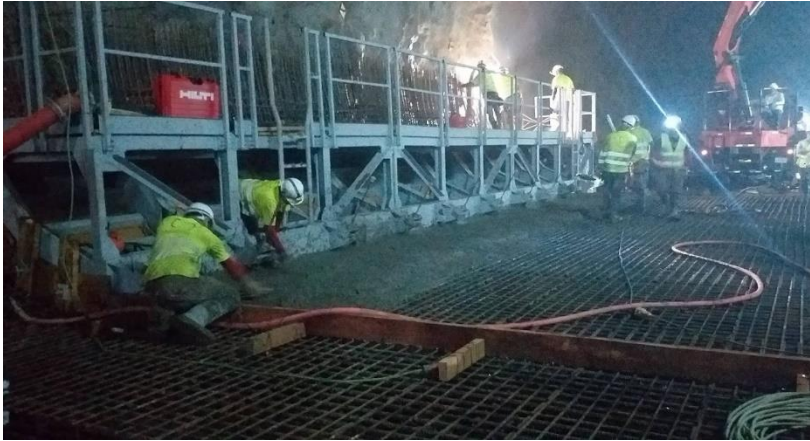
Construction of upstream permanent invert slab
