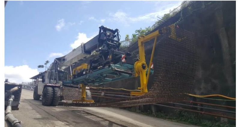
Transporting reinforcement cages into tunnel for construction of invert upstream and downstream
