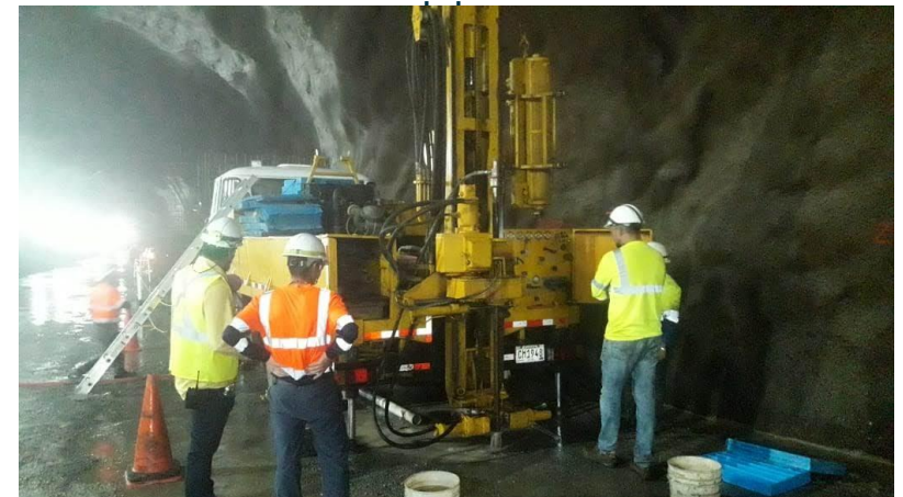
Coring Investigation to verify lining design
