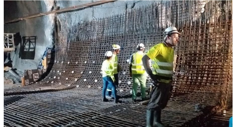
Construction of downstream permanent invert
